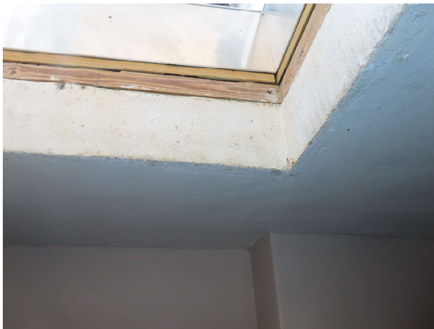
Structural concrete roof deck
